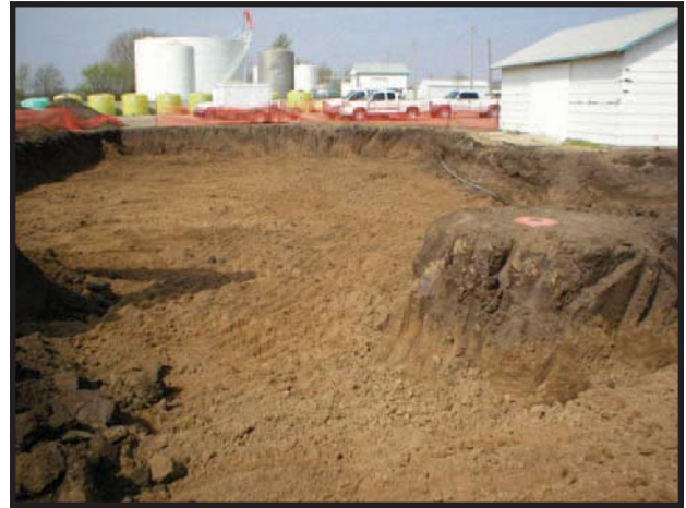
A primary emphasis for cleanup of agricultural facilities is source removal.
