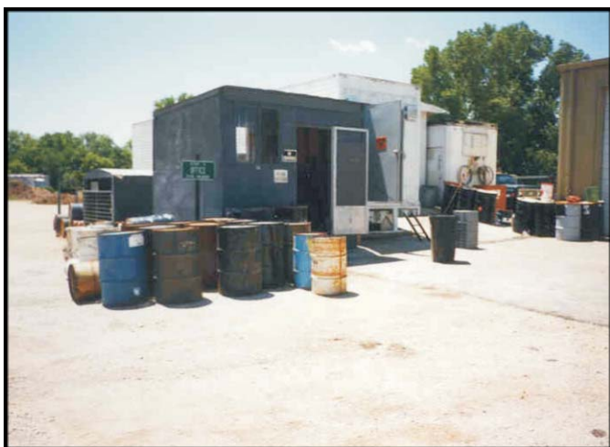
Household hazardous waste building.
