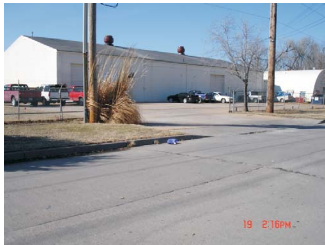
View of Dawson Brothers, Inc., facility.
