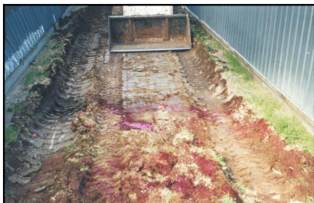
Stained soil prior to excavation.
