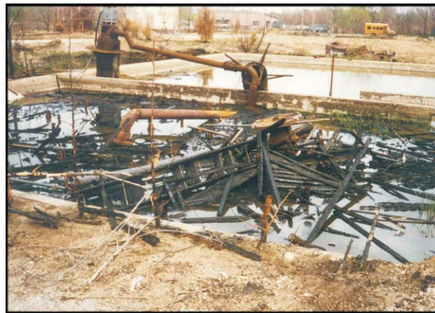
Storm water collection pits.
