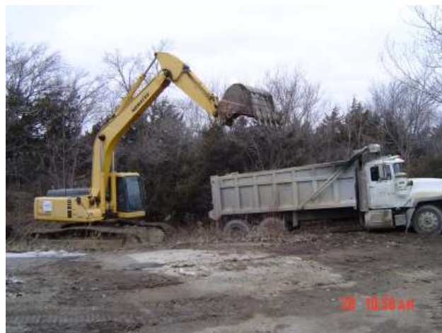
A trackhoe removes contaminated soil from the lagoon area.
