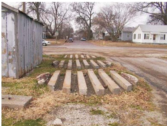
The BTA Property as seen from the northeast corner
