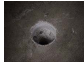
Figure 2. Drilled hole for subslab port
