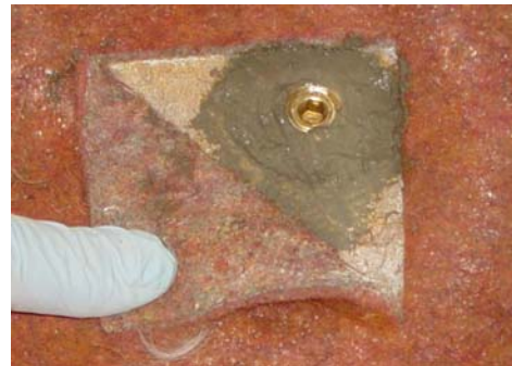
Figure 3. Completed subslab port
