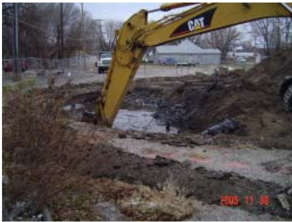
Removing the contents of the gas holder tank at the former manufactured gas plant in Manhattan. The contents are primarily water, woody debris, soil, and hard-parts refuse.
