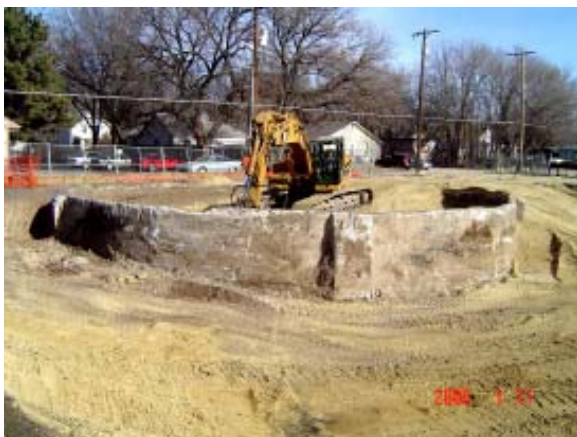
Filling the gas holder with clean fill. The bottom of the gas holder tank was broken to prevent water from continuing to collect in it.
